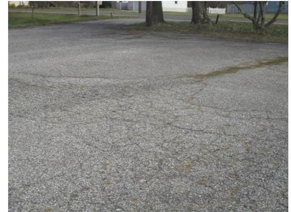
Off of the southwest corner of the building there is a downspout that could be redirected into a downspout planter box to reuse roof runoff. At the time of the assessment the parking lot was in poor condition. When it comes time to repave, parking spaces can be replaced with pervious pavement to capture and infiltrate stormwater. A preliminary soil assessment suggests that the soils have suitable drainage characteristics for green infrastructure.
