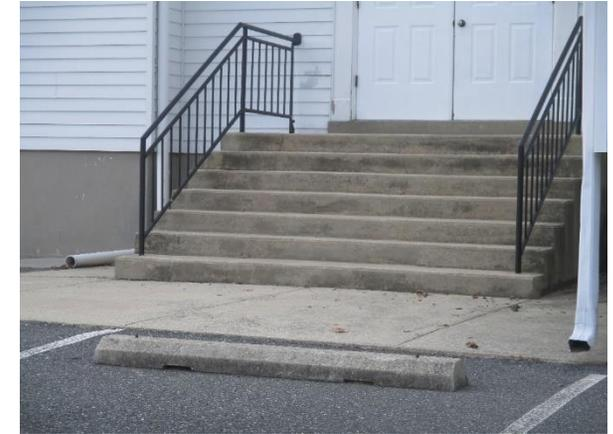
There are multiple downspouts that release rainwater onto the parking lot. Parking spaces can be replaced with pervious pavement to capture and infiltrate stormwater as well as help alleviate the erosion that is occurring across the street. A preliminary soil assessment suggests that the soils have suitable drainage characteristics for green infrastructure.
