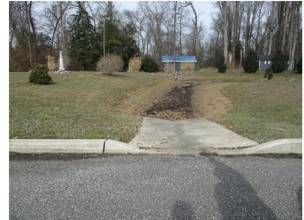
The existing swale that is functioning as a non-natural conduit is conveying water from the parking lot to a turfgrass area. The existing conduit can be converted to a bioswale to prompt groundwater recharge and enhance aesthetics. A preliminary soil assessment suggests that the soils have suitable drainage characteristics for green infrastructure.
